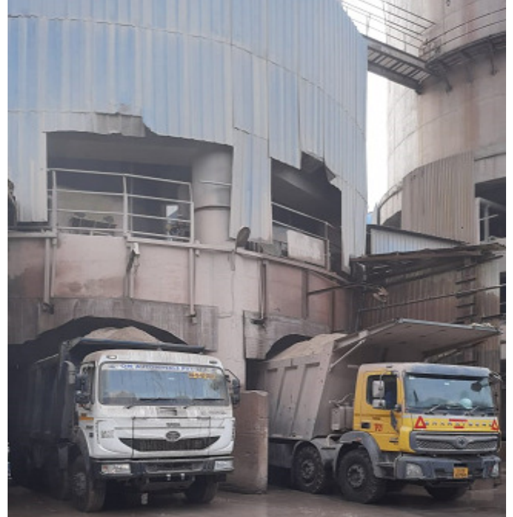
Figure 2 Flyash storage Silo
