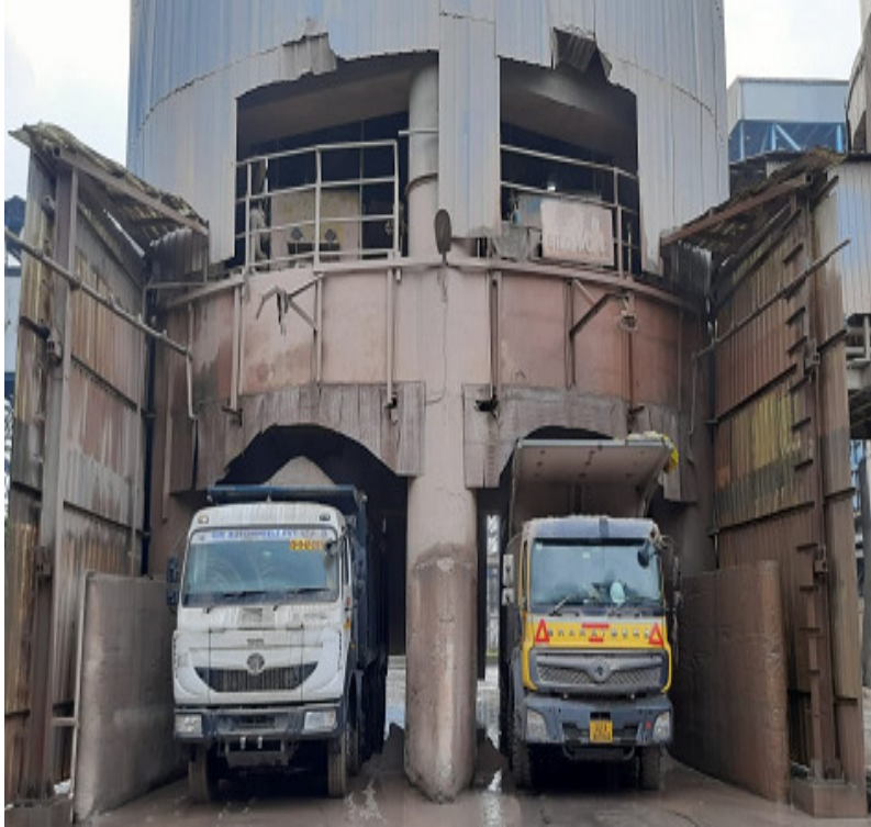
Figure 1 Flyash storage Silo
