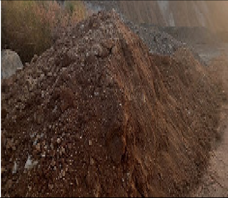
Figure 3 Fly Ash dosing and compacting using overburden and Soil
