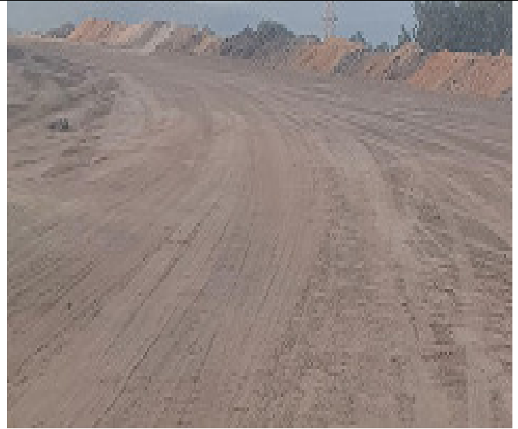
Figure 4 Fly Ash dosing and compacting using overburden and Soil
