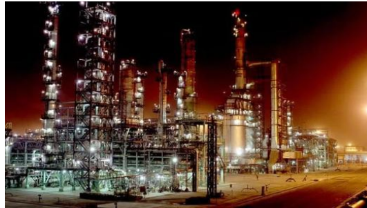
IOCL Gujarat Refinery
