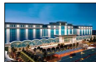
Prayagraj Railway Station Re- Development
