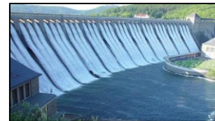
Ratle Hydroelectric Power Project
