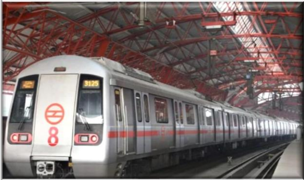
Delhi Metro Rail Corporation (DMRC)
