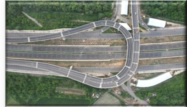
Urban Extension Road II
